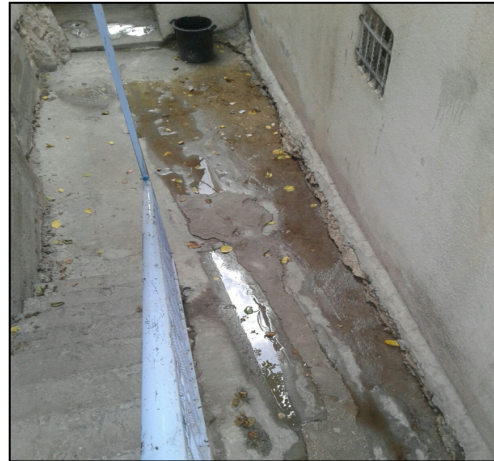
Picture 2. Sewerage critical point
