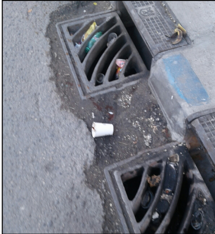
Picture 1. Drainage critical point
