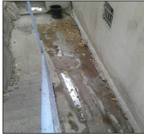
Picture 2. Sewerage critical point
