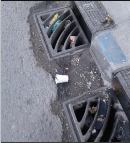
Picture 1. Drainage critical point
